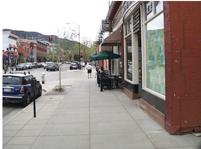
concrete walk surfaces with scoring
