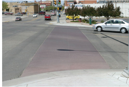
existing colored concrete crosswalk in Casper
