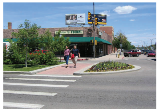
median island at intersection
