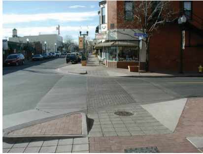
concrete paving corner ramps
