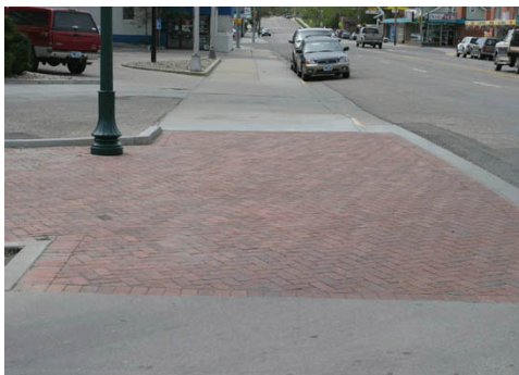
existing bikeway paving at an intersection
