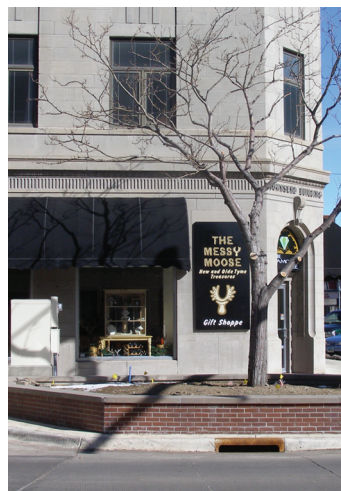
existing concrete planter at Second Street
