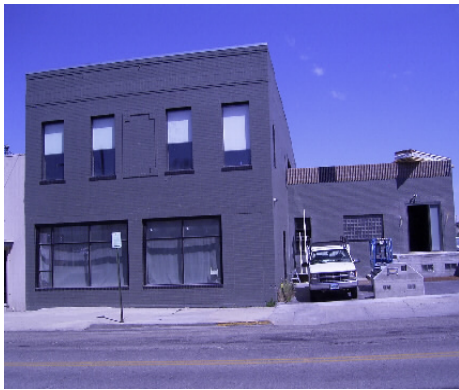
Shawn and Shane Rivett have done a marvelous job at turning the former Wyoming Stationery building into a beautiful residential loft. They opened up their home for a tour spotlighting the Old Yellowstone District and Civic Auditorium projects in early March. What a wonderful treat!
