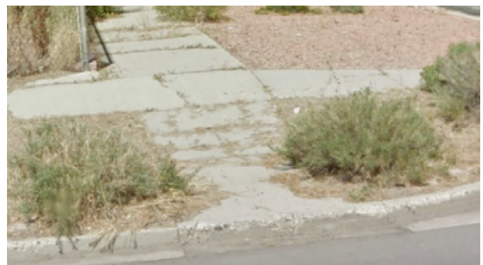
Figure 3-23 – Example of Substandard ADA Sidewalk Sideslope
