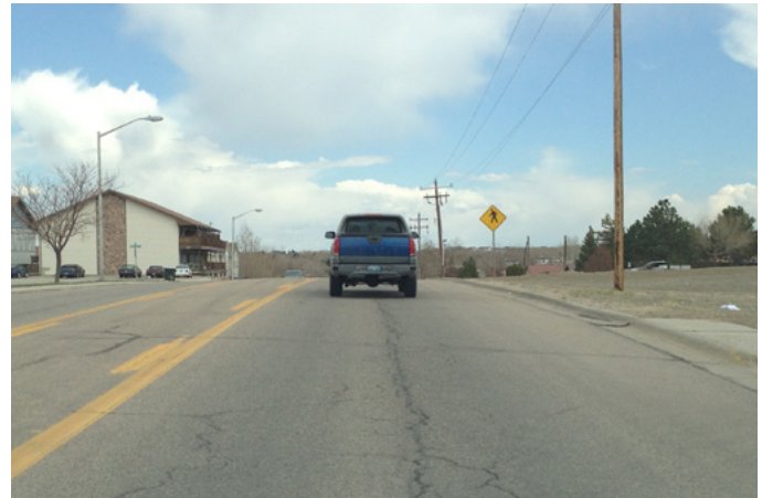
Figure 3-31 – Example of Longitudinal Cracking in Study Area
