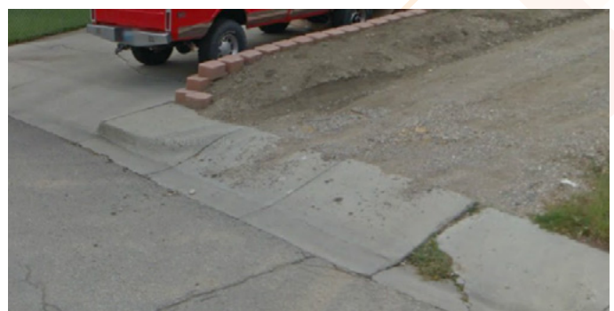
Figure 3-23 – Example of Substandard ADA Sidewalk Sideslope
